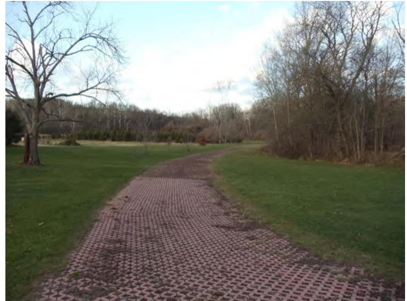
View of permeable drive with additional Township-owned land in the distance.
