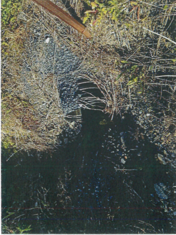
Photo 17 – Outfall 12 – 18-inch N-12 plastic pipe leading to headwater wetlands of Dry Run.
