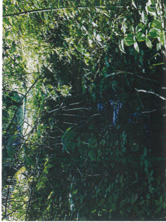
Photo 22 – Outfall 16 – 18-inch reinforced concrete pipe to Hokendaqua Creek.
